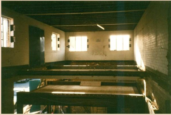
The garage originally had very high ceilings to accommodate the fire tenders so the upper level floor was lowered, and became the General Store with the Sensitive Store at the far end.
